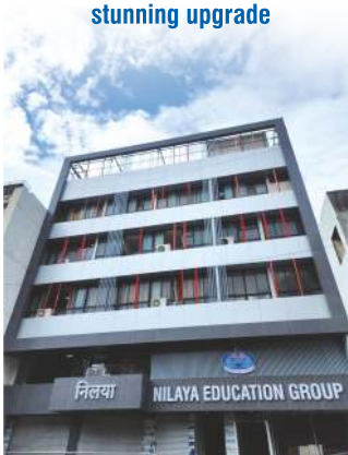
7 Storage Huge Building
